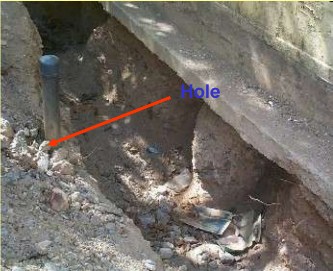
Hole for GPR investigation Edificio Royal
