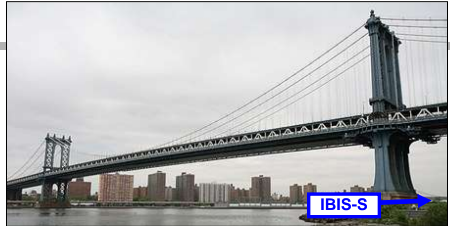
BRIDGE SIDE VIEW
