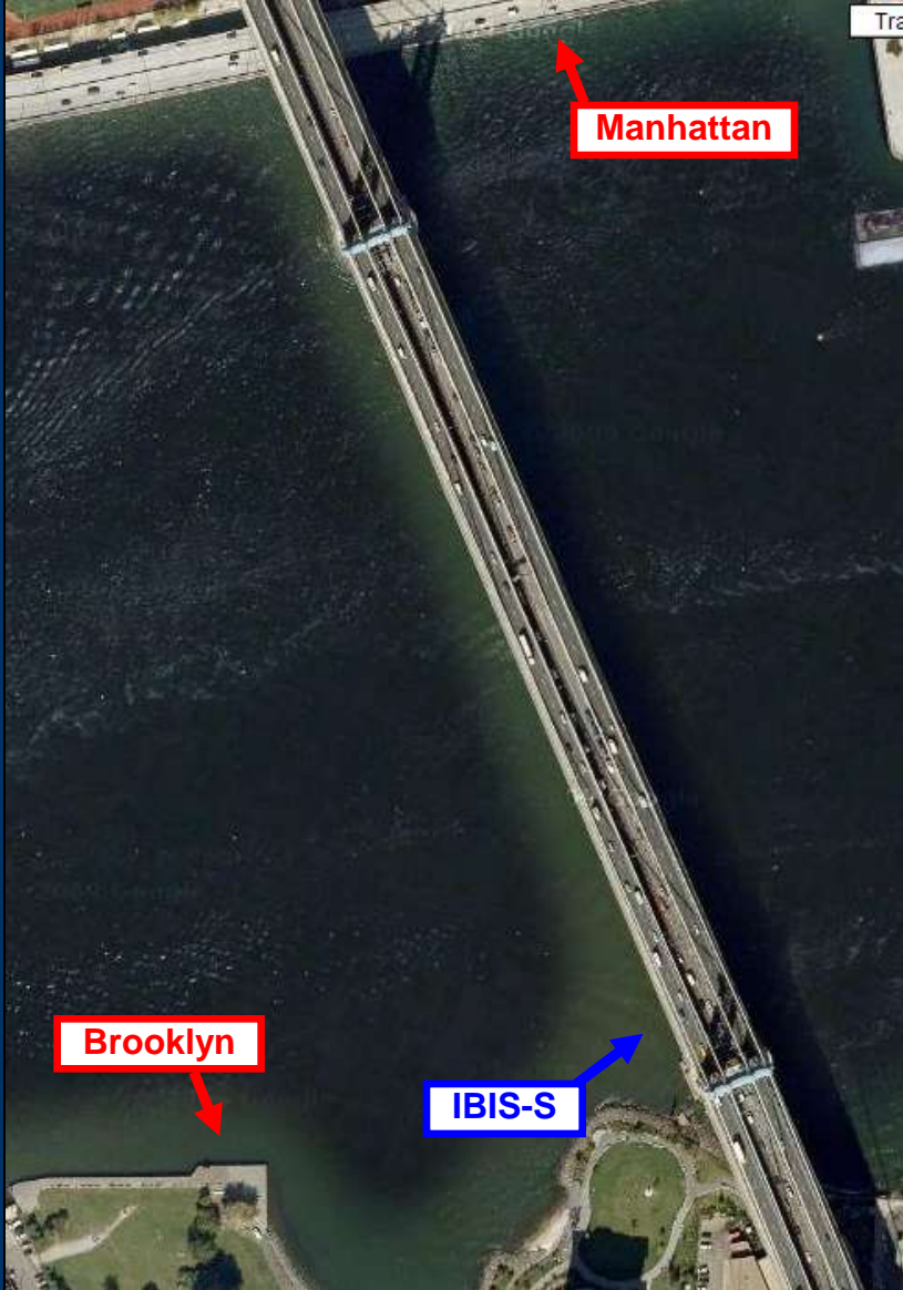
BRIDGE TOP VIEW
