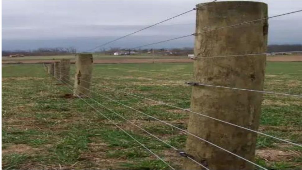
Figure 8. High tensile eight wire fence [46]
