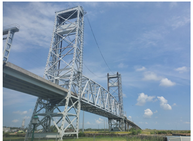
Figure 1. Ellender Ferry Bridge, SR 27, Calcasieu Parish, Louisiana
