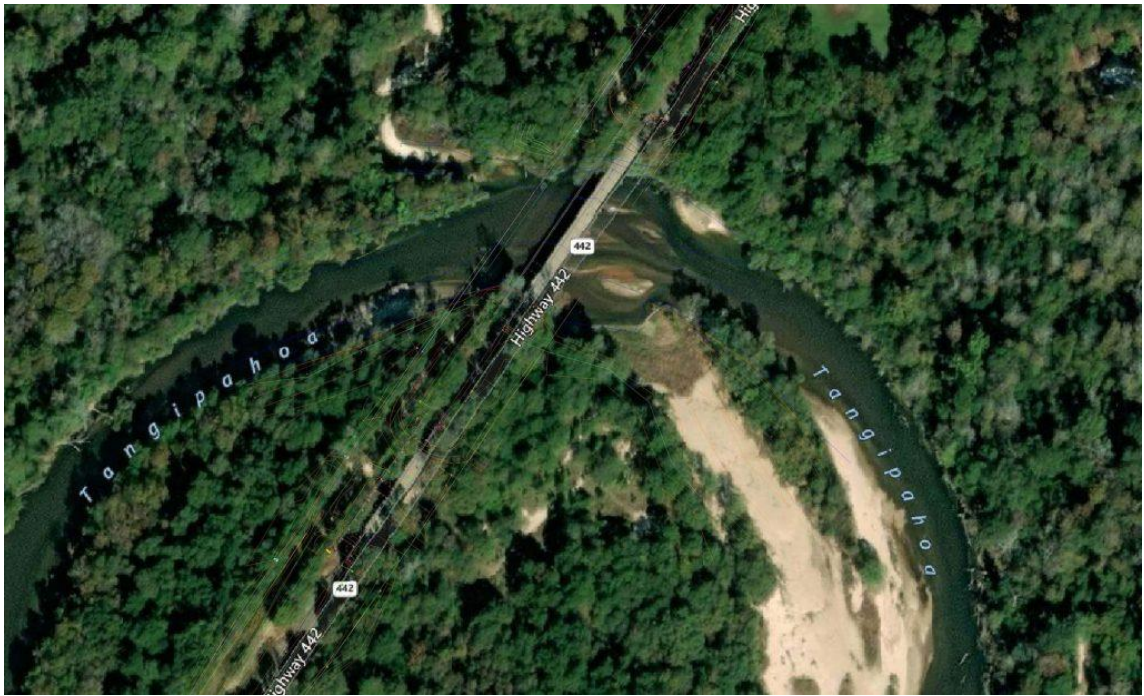
Figure 42. Location of Tangipahoa River Bridge
