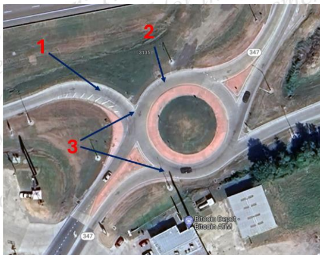
Figure 51. Possible reasons for hotspots at Interchange 8
