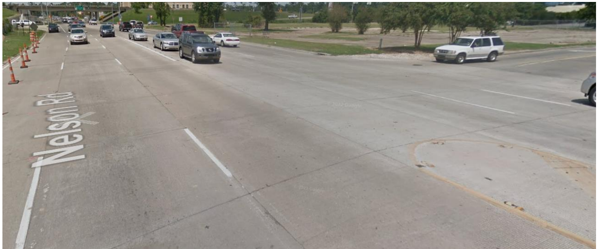
Figure 14. Raised Curb Channelization (Nelson Road - 30.195263, -93.249429) Pre-Treatment
