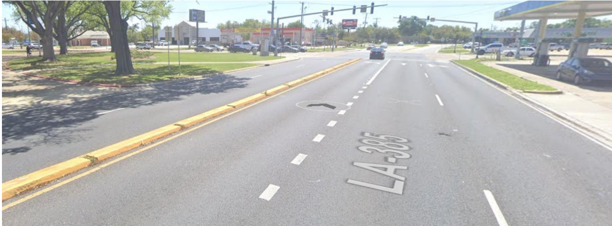
Figure 9. Raised Median (Ryan Street - 30.176669, -93.218558) Post-Treatment
