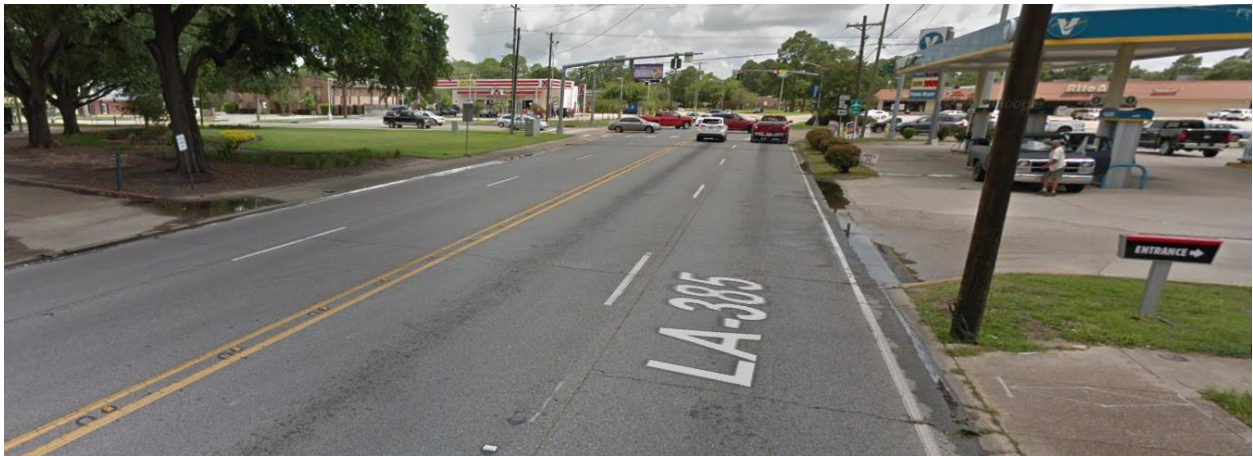
Figure 8. Raised Median (Ryan Street - 30.176669, -93.218558) Pre-Treatment
