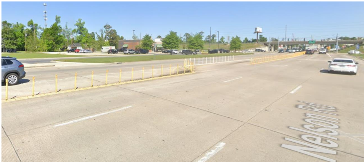
Figure 15. Raised Curb Channelization (Nelson Road - 30.195263, -93.249429) Post-Treatment
