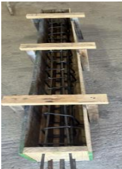
(a) Reinforced concrete mold for casting beams
